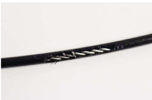
A TEAR IN THE CABLE COVER
