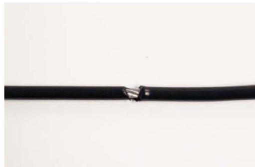
A CRACK IN THE CABLE COVER
