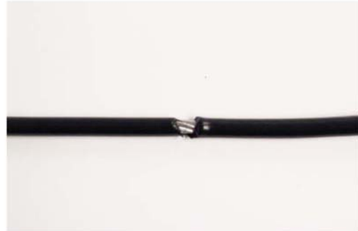
A CRACK IN THE CABLE COVER
